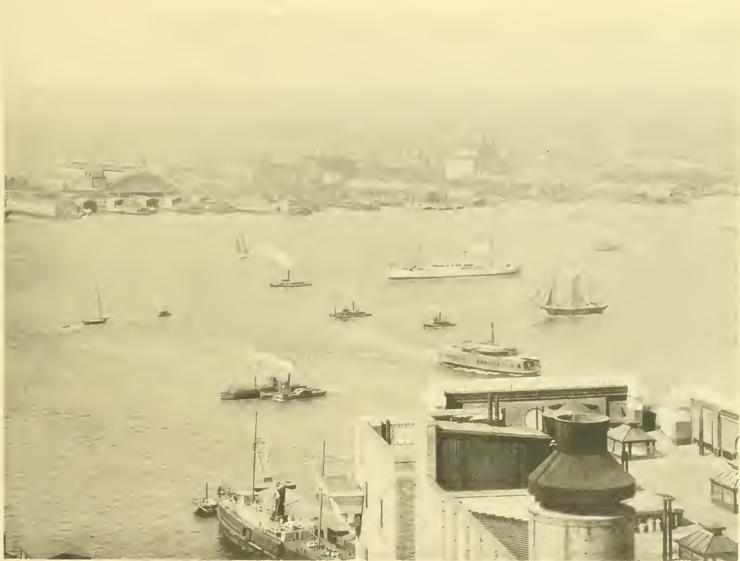
HUDSON RIVER AND JERSEY CITY from Bowling Green Building.
